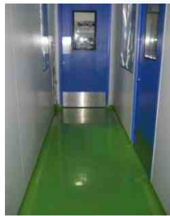
DOORS & EPOXY FLOORING
